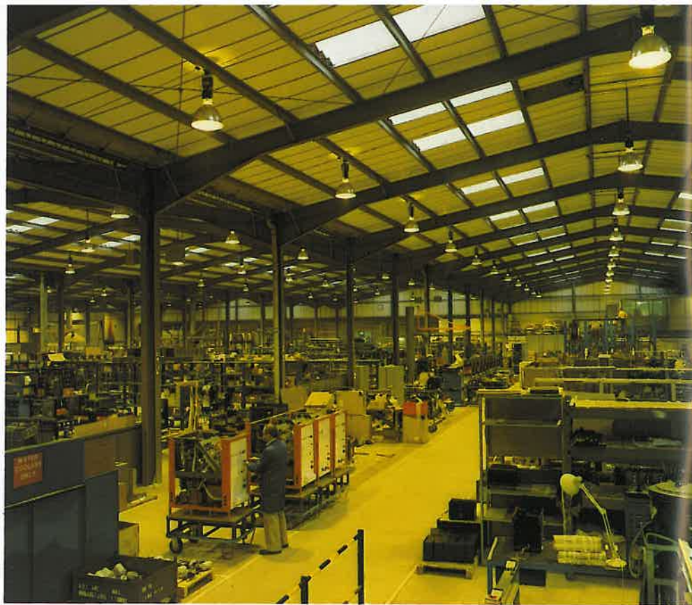
The British Oxygen Company's factory at Ramsgate, Kent is lighted by 204, 250W SON lamps in Hi-Pak fittings, and was commissioned in August 1977. Only four lamps have failed since installation, in nearly 18,000 hours use.
