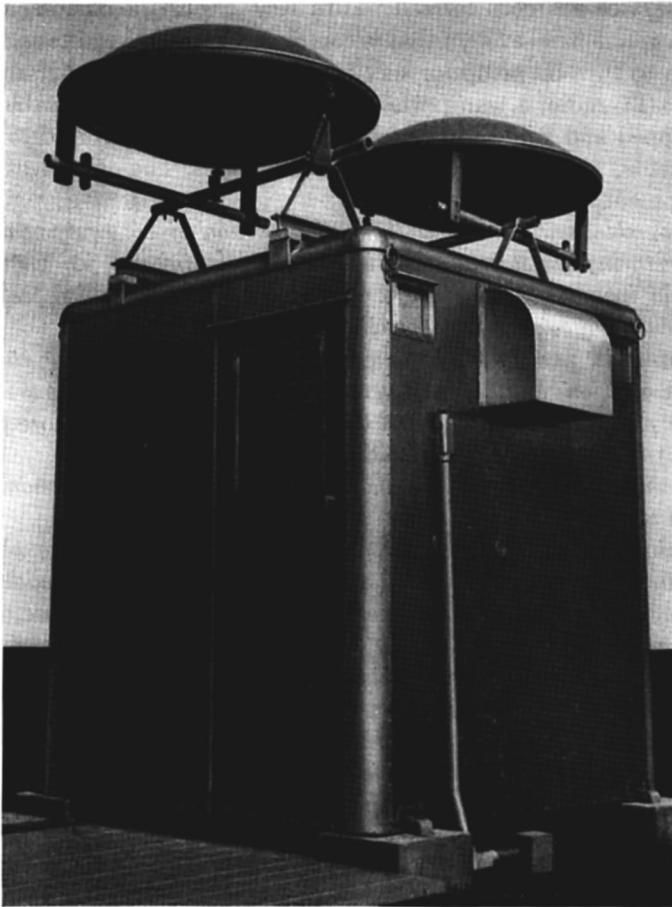
Fig. 41 — 7-foot \times 7-foot shelter equipped with two 5-foot paraboloidal antennas.
