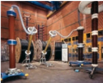
High voltage laboratory, partial discharge measurement and ac voltage test
