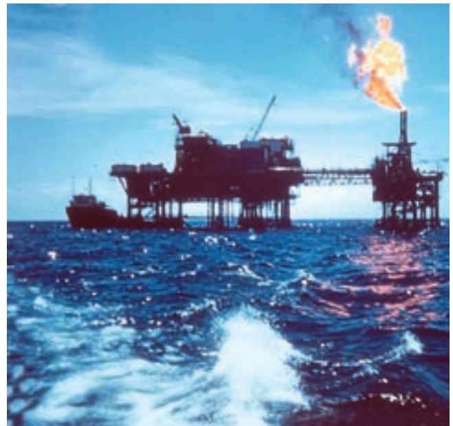
Offshore production platform in Indonesia, with power supply through a submarine cable
