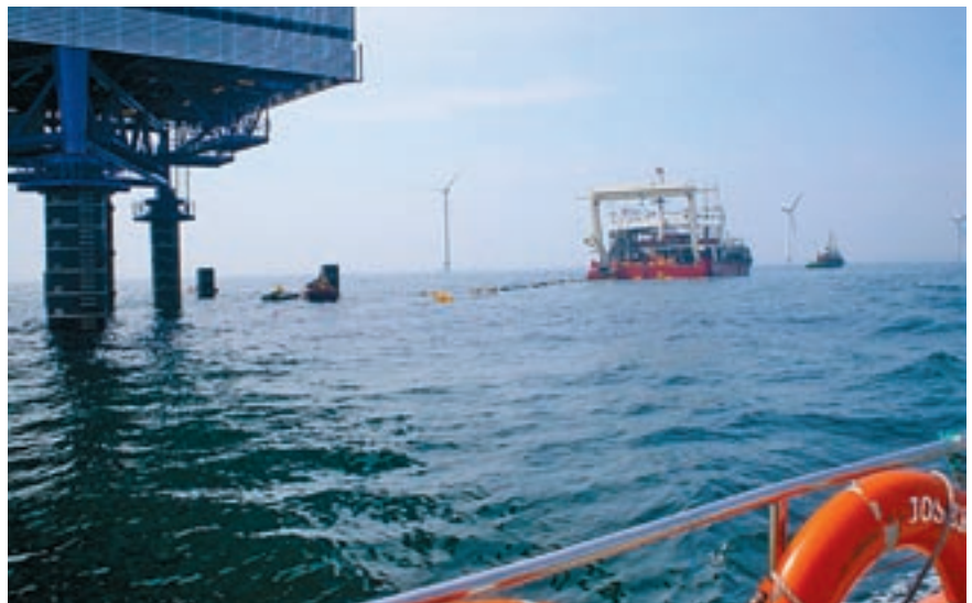
Cable laying within an offshore windfarm
