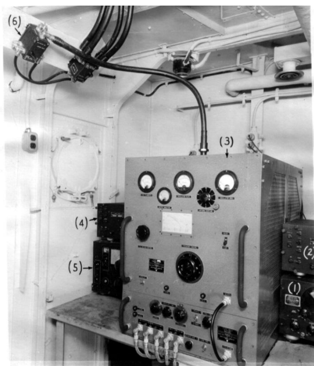
F644C5506 NAVY YARD, NEW YORK JANUARY 14, 1944 U.S.S. DD 427. (1) RBK RECEIVER. (2) RBW PANORAMIC ADAPTER. (3) XCJ-1 TRANSMITTER. (4) RCX PANORAMIC ADAPTER. (5) RAO RECEIVER. (6) TRANSMITTING ANTENNA SWITCHES.
