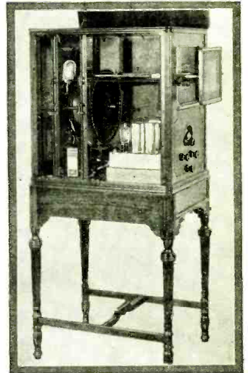
Side-view of new home projector with Crater lamp and lens disc.
