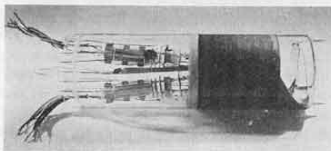
Fig. 10—Single sided target, electrostatic deflection Graphechon.
